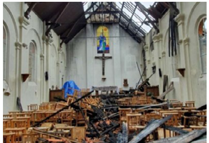
The aftermath of an arson attack at a church in France, 4 July 2020. (OIDAC)
