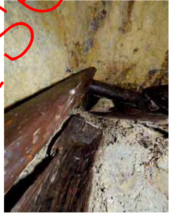
Launder (wooden water-channel) that received water from the still adjacent remains of the upper waterwheel in Cătălina Monulești Mine. (© C. Tamas)
