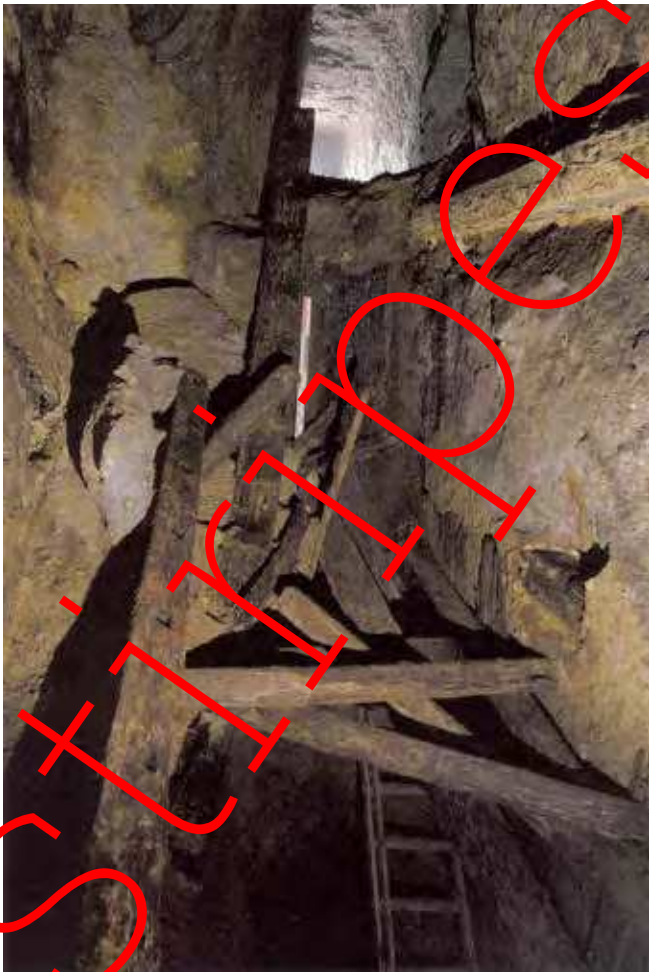
Păru Carpeni: Water wheel chamber with monoxyle ladder - as discovered in situ. (© B. Cauuet)
